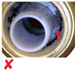
Dirt/debris inside fitting
